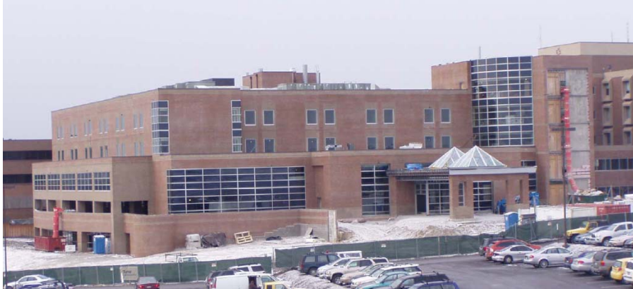
Photograph 1: Monongalia General Hospital from South-East, During Construction
